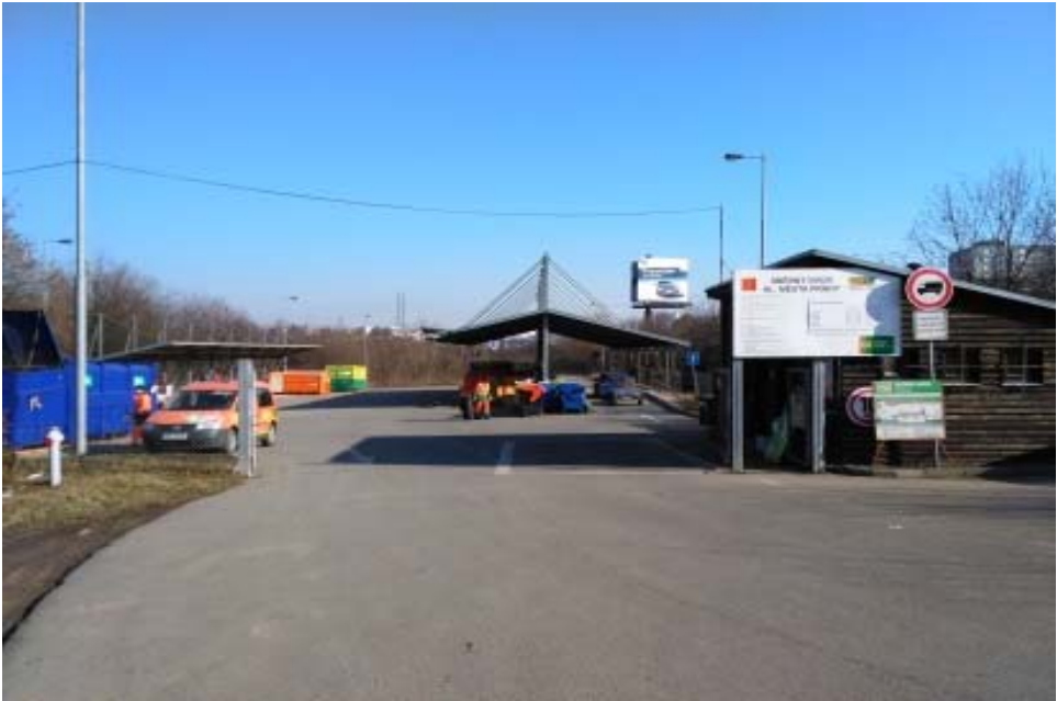
Figure 4: Civic amenity site on the street Zakrytá in Prague 4
